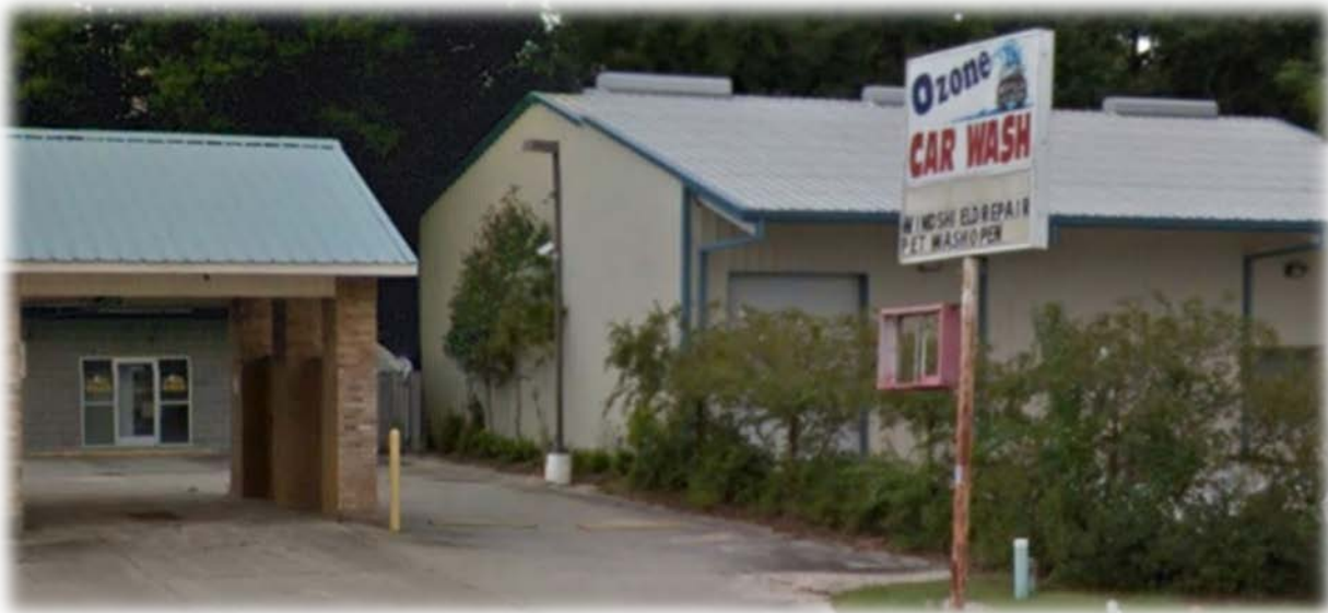
Ozone Car Wash in Covington, courtesy Google StreetView
